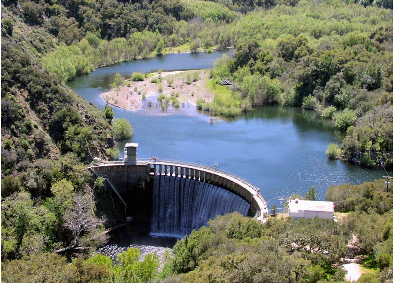
San Clemente Dam on the Carmel River is about 90% full of sediment.
