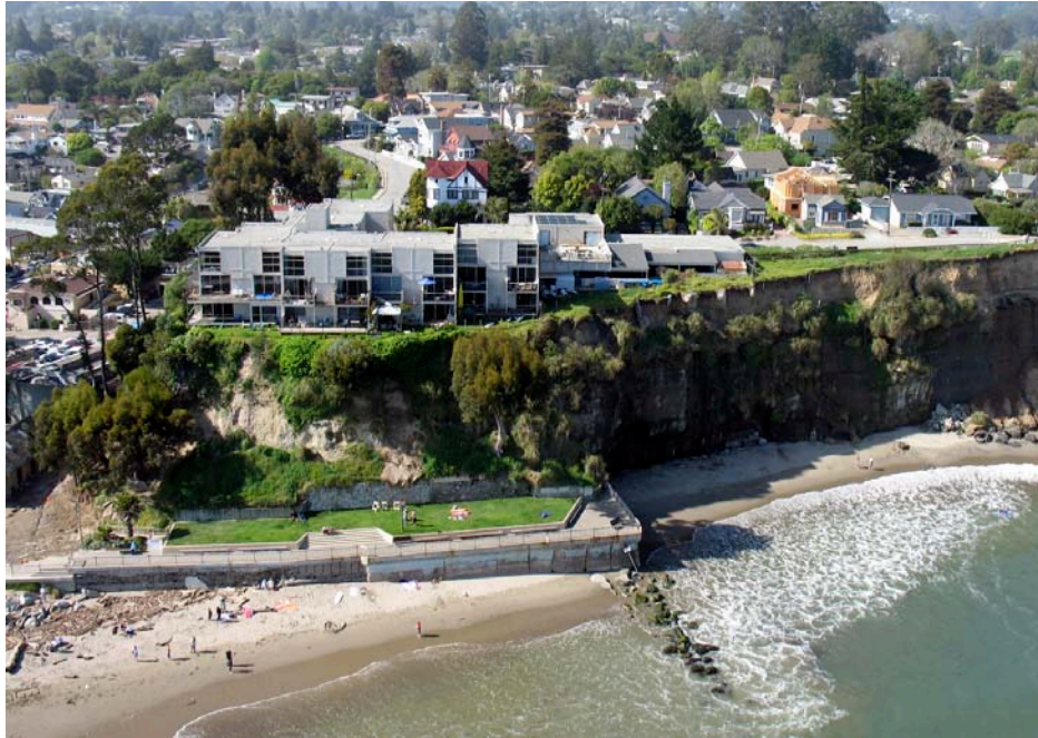
This rock and concrete seawall built to protect the sewage pumping station in Capitola was built over 80 years ago.
