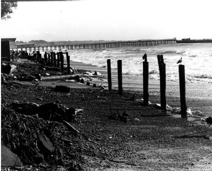
*The timber seawall at Seacliff State Beach has been built, destroyed by wave and rebuilt eight times over the past 80 years.*
