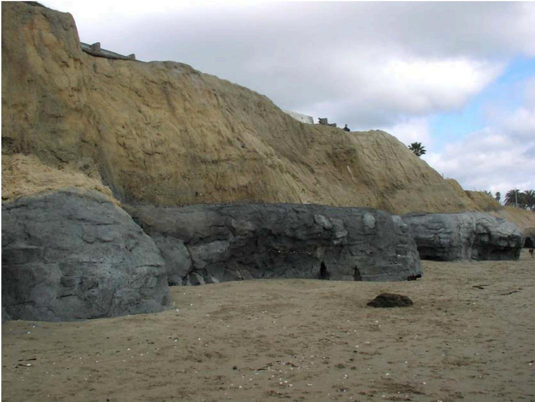
*A soil nail wall consisting of shotcrete or gunite textured and colored to match the natural rock was used to stabilize the cliffs along Pleasure Point.*
