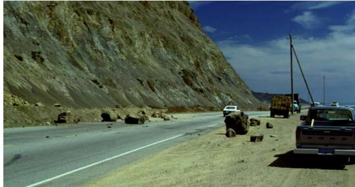
*This 1978 photograph shows one of the rock falls on Highway One at Waddell Bluffs that made it through the trench that was designed to catch the rocks.*
