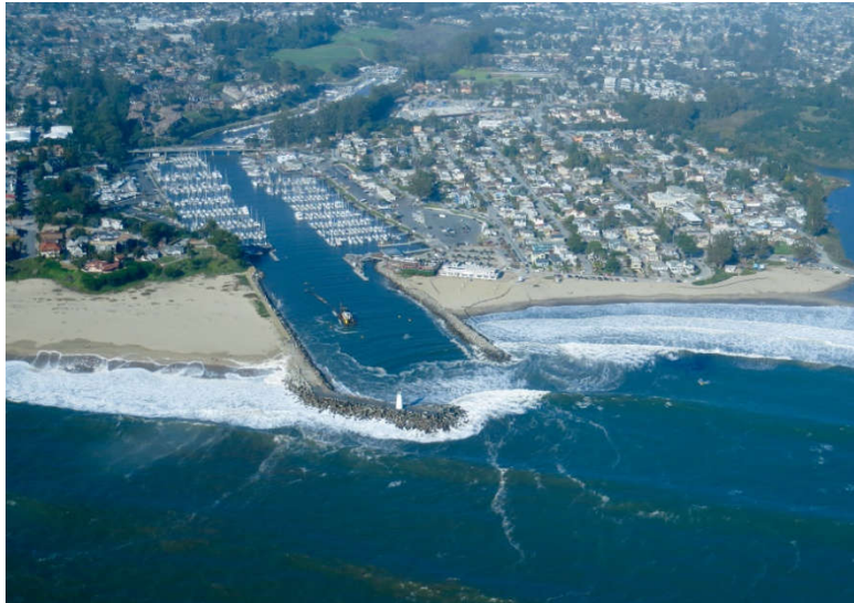
The dredge in the harbor entrance.
